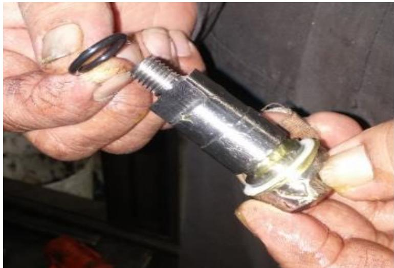
8. Insert the **BV Stem Assembly** into the "through hole" of the **BV Body** until fully engaged.
